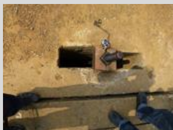
Padlocked sluice gate
