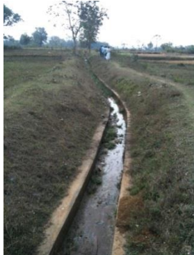
(c) Well-built farmer-constructed canal lining, OCTMP, Odisha.
