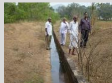
WUA Executive Committee members inspect the concrete lined Main Canal
