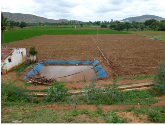
(g) Combination of borewell and in-field storage reservoir. Water is pumped into the lined reservoir from the borehole and distributed by gravity irrigation to the plots, KCBTMP, Karnataka
