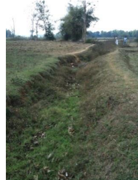
(d) Unlined canal section at tail of the same system. No uniform shape, high seepage losses and unable to maintain command at outlets, OCTMP, Odisha.
