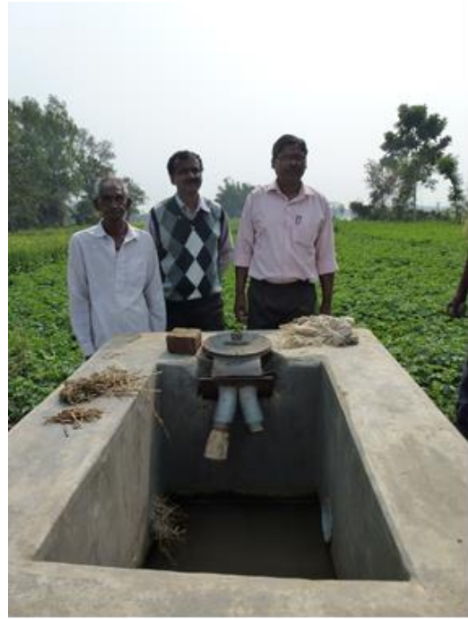
(b) Spout outlet into a chamber, which the farmers have adapted to provide two connections for lay flat pipes, Naskarpur Ghantipara Mini RLI scheme, West Bengal
