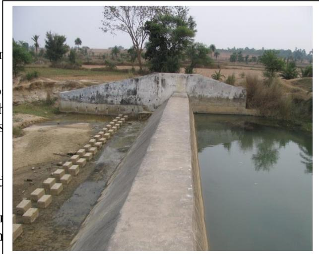
To facilitate smooth flow of approaching floodwaters towards the weir, the upstream area of the weir is cleared for the required width and to the levels, to prevent heading up of water that may cause overtopping of the embankment.
